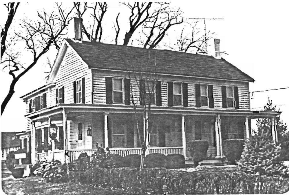
House (A): View North
