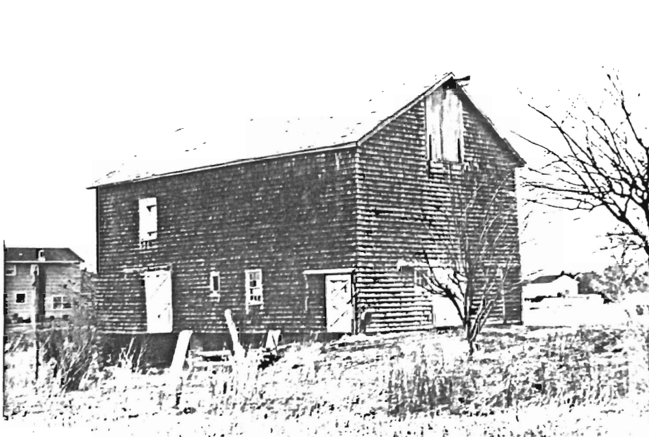
Barn (C): View NW
