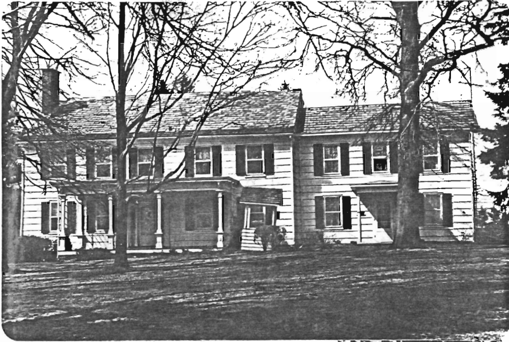
House (A); View North
