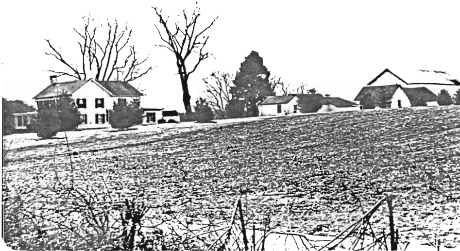
Complex; View West
