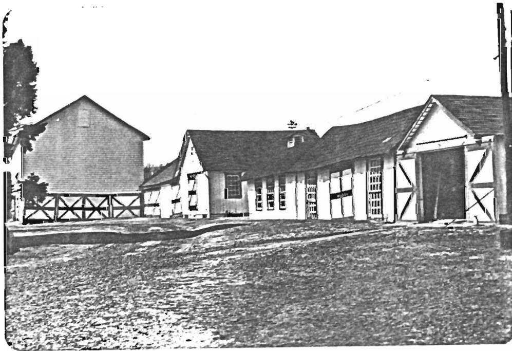
Sheds (C); View North
