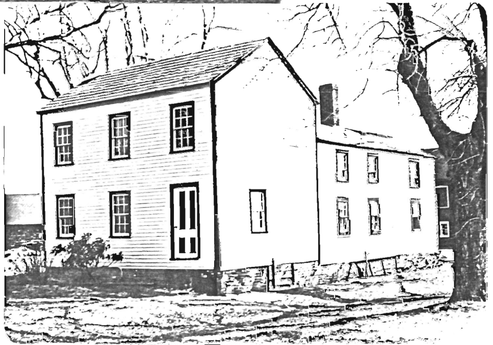
House (A): View SE
