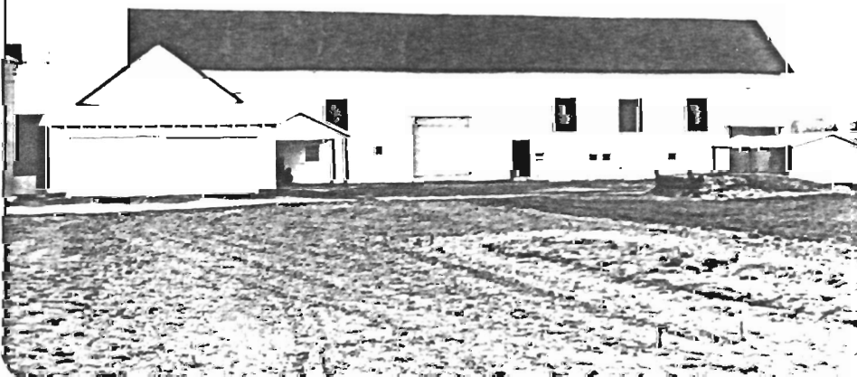
Barn (B); View North
