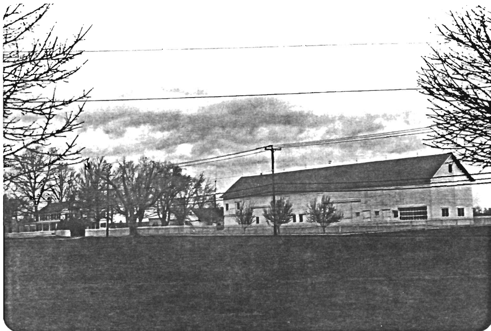
Complex; View West
