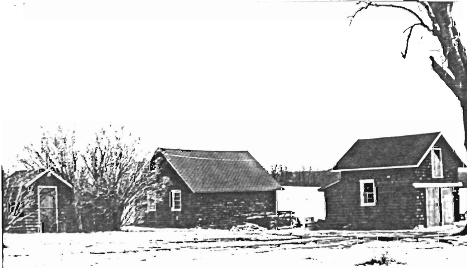
Sheds (C): View SE
