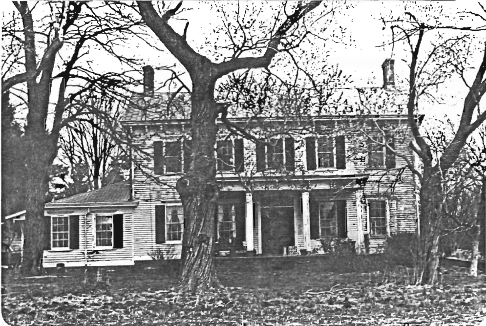
House (A); View North
