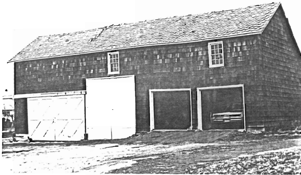
Wagon/Equipment Shed (B): View NW
