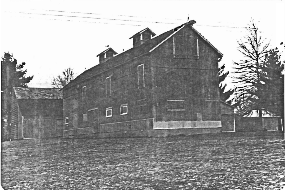
Barn (C): View Northeast
