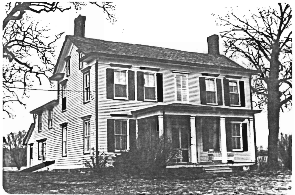
House (A): View NE
