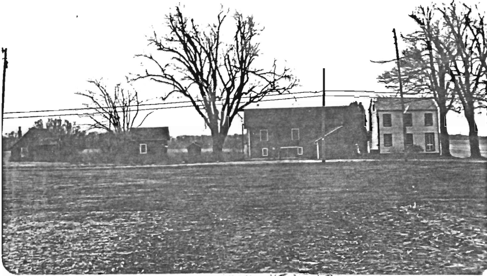
General View of Complex; View South
