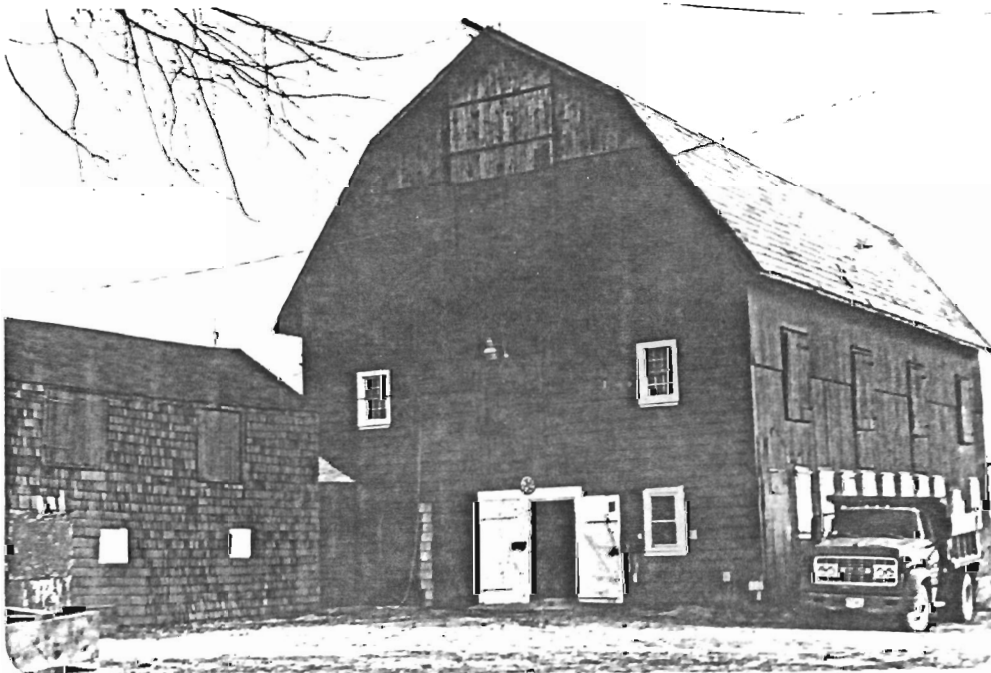
Barn (C); View SE
